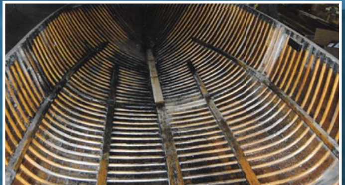
Interior gutted before sanding and finishing
