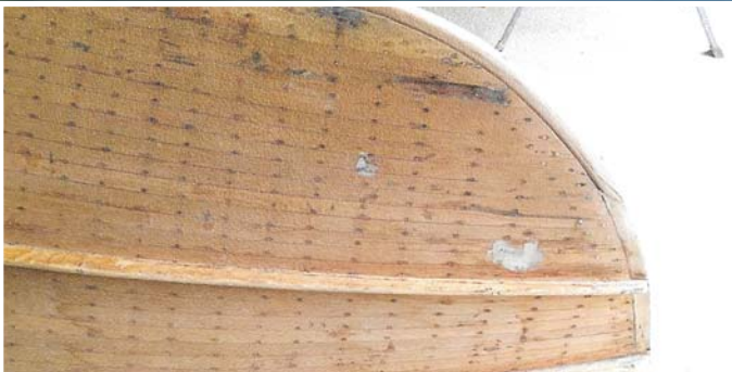
Replacing the full stem
